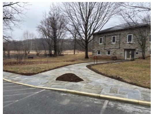
Gambrill Mill Rehabilitated Sidewalk
