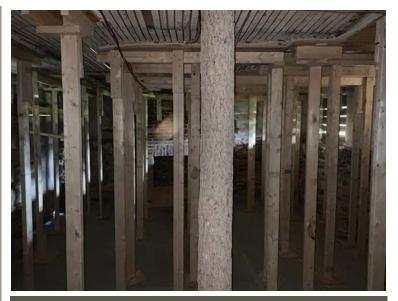
Modern 2x4 supports surround a historic log support in the basement of Worthington House. The modern framing secures the historic plaster snuggly against the lathe so specialists can rekey it by pouring a plaster slurry on it from above. Prior to the stabilization of the ceiling plaster in the Worthington basement, visitors were limited to standing near the doorway during open house tours and therefore unable to look out the cellar window as young Glenn Worthington had during the battle.
