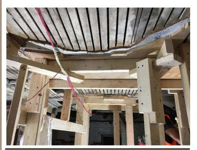
Preservation specialists use a variety of techniques to stabilize and preserve the original plaster in the Worthington basement. Wood supports close the gaps between the plaster and the lathe. Anchors help secure the plaster in place. Edges are smoothed and sealed to prevent moisture infiltration and future damage. Finally, a slurry of plaster will be poured from above to rekey the plaster to the lathe.
