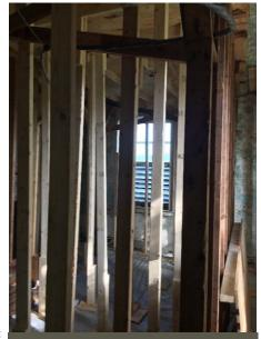
Structural and temporary bracing on the first floor of the Best House. Preservationists restructured the bracing in the Best House to allow visitors better access during open house tours. Temporary bracing was used to hold historic plaster in place while it was repaired and reattched to the lathe.
